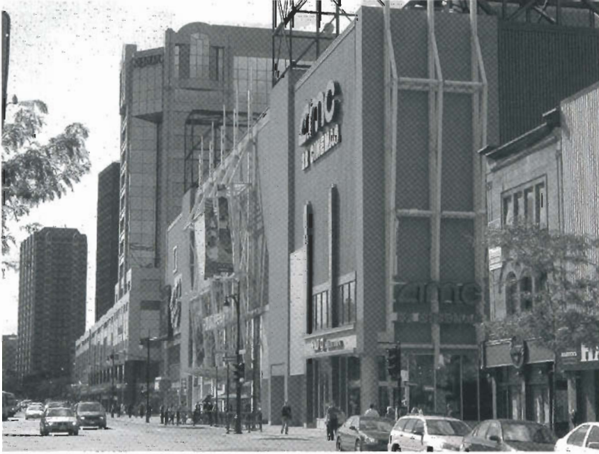
FIGURE 2 A STREET VIEW OF THE FORUM ENTERTAINMENT CENTER (FOREGROUND) WITH THE SHOPPING CENTER AT REAR.
